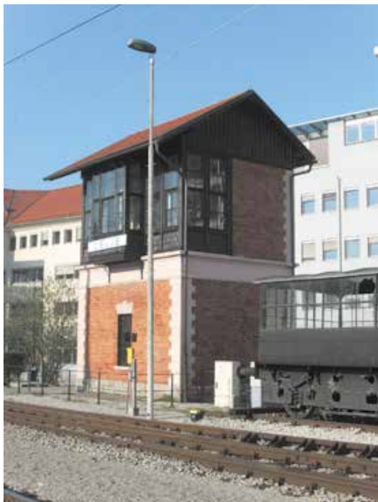
Figure 9: The Number II Signal Box in Celje was built between 1906 and 1909. A tower-like masonry structure almost 10 metres high, it had a wooden viewing platform and was equipped with points machinery that was used to remotely operate points and signals. It is the only surviving example of a signal box of this type anywhere on the Vienna - Trieste railway line (photo: Damir Žerič).
