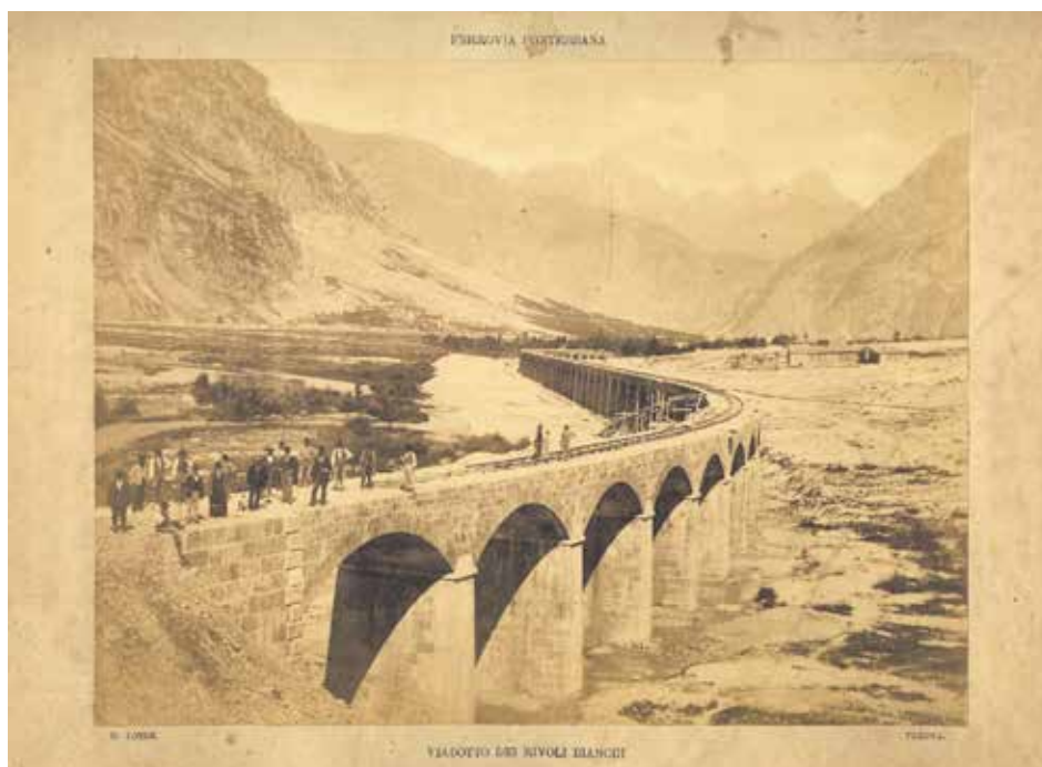
Figure 6: Rivoli Bianchi viaduct under construction along the «Pontebbana» railway. Photo of the Lotze studio, Verona, 1876 (Biblioteca Vescovile di Rovigo)
